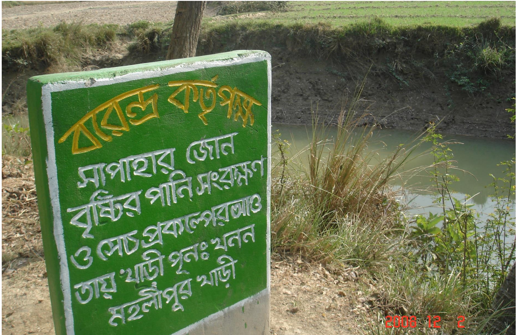
Re-excavation of natural canal (Khari) for supplementary irrigation in Kharif-II and early rabi season
